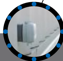
Exterior receptacle covers
